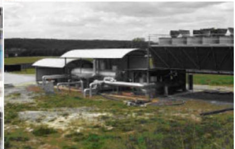
Series 250 Containerized ORMAT Energy Converter Power Unit
