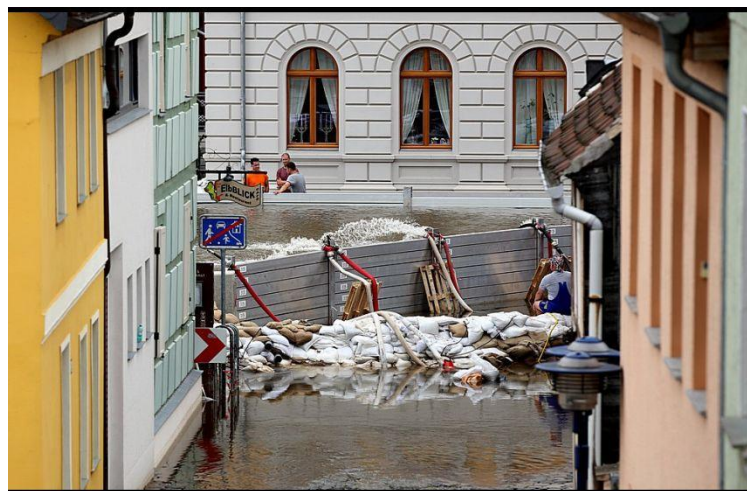
Figure 4 . Facilities for fighting floods in urban conditions
