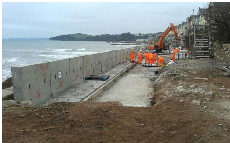
Figure 3. Constructions erection aiming at high water protection
